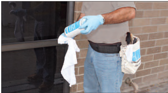
The Correct method is to pour on the cleaner. Dipping the rag into the solvent is incorrect, as this will contaminate the cleaning agent.
